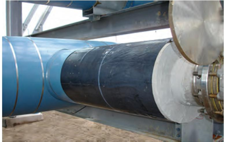
Vapor retarder mastic coating over ISO-C1 at termination. Aluminum jacket adds mechanical protection to the insulation system.
