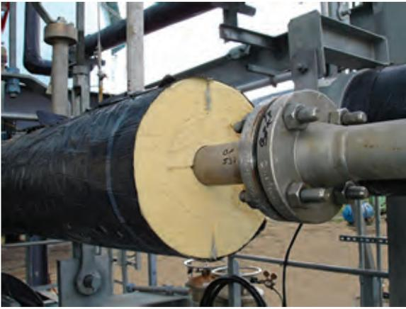
Staggered, double-layer ISO-C1 polyiso, terminating at flange. Joint sealant on outer longitudinal seam; vapor retarder sheet.
